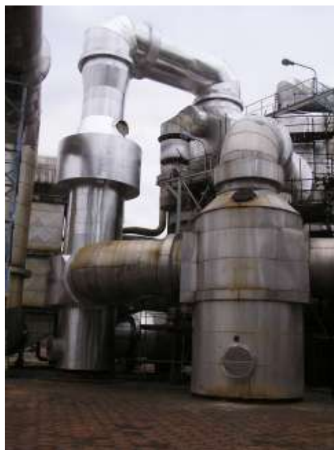
Heat exchangers VT1, VT2
